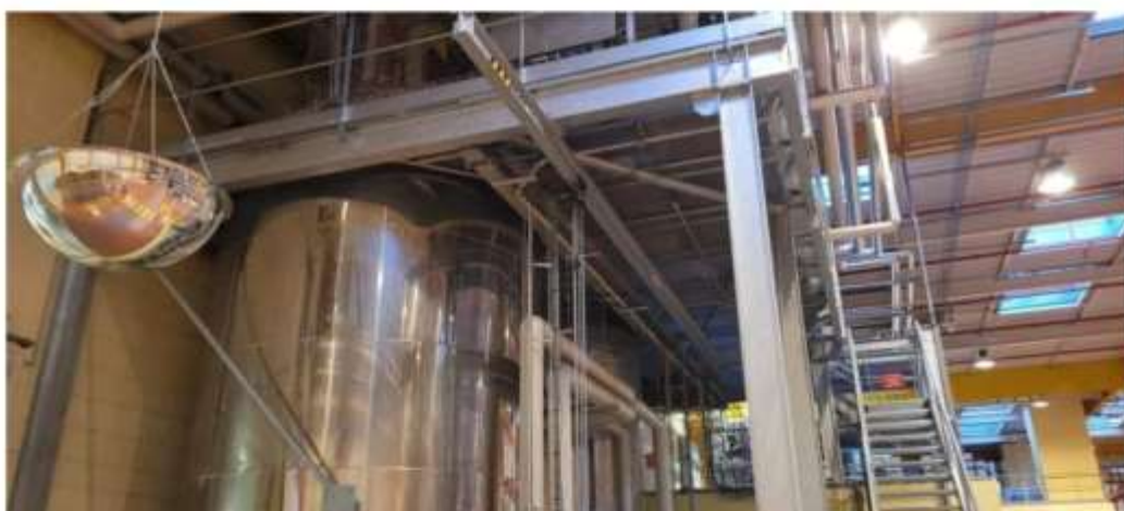
Manut Services installs monorail and Verlinde VHR 2 chain hoist
